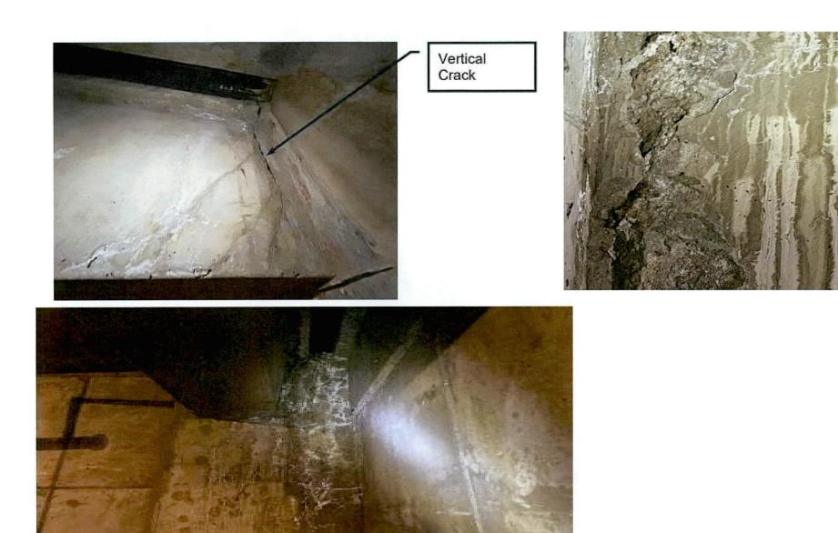
Mineral Deposits on the face of the concrete indicate significant water intrusion.
