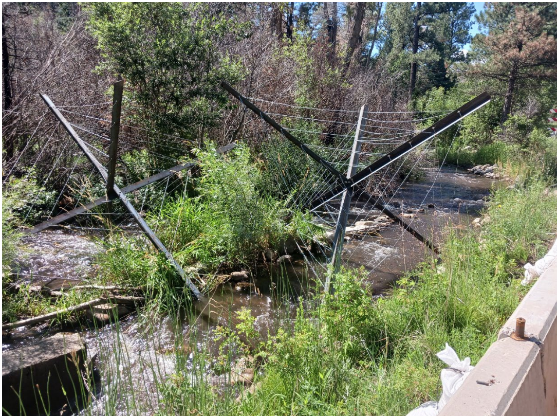
Burn Scar Flooding Mitigation Jacks in Mora County
