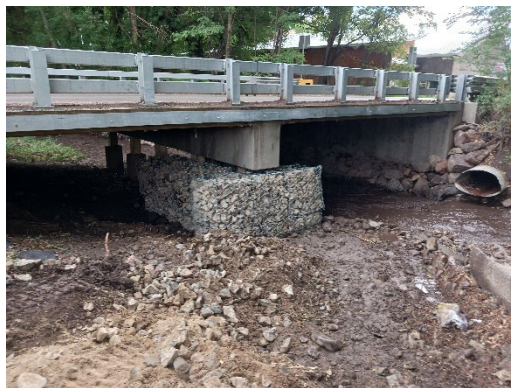
Gabion Basket Mitigation Protects a Bridge Structure
