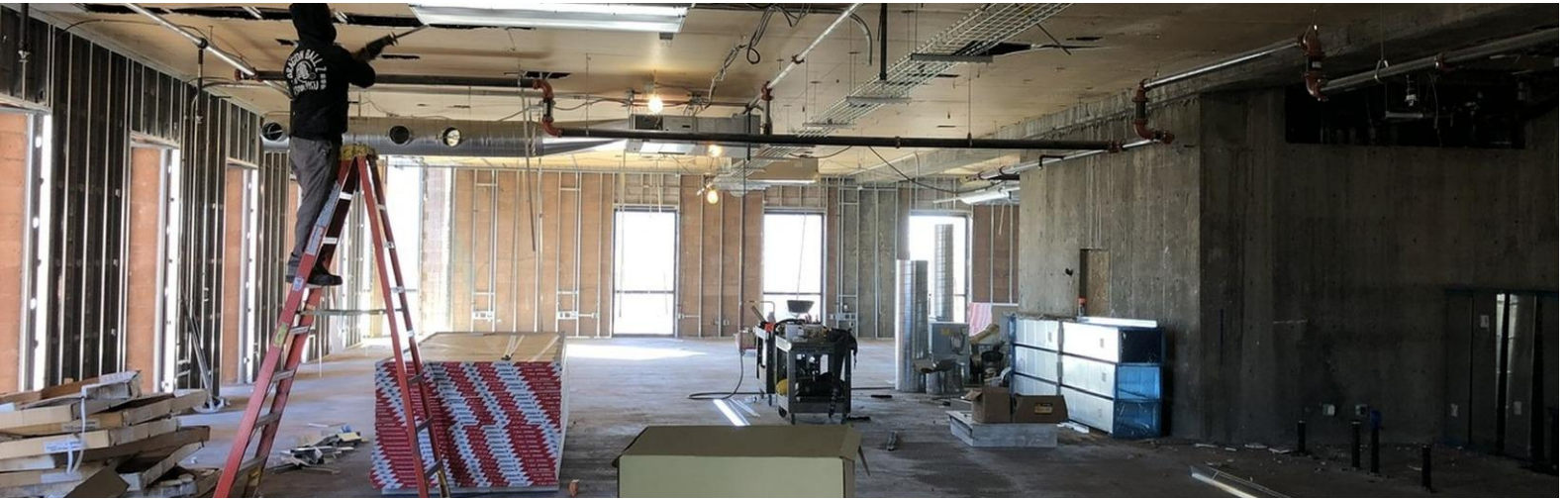
Mechanical Work delivered under an Energy Service Performance Contract.
