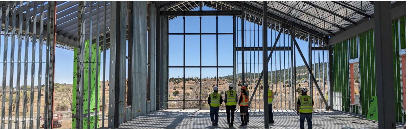
The New Mexico Behavioral Health Institute Project in Las Vegas is currently under construction.
