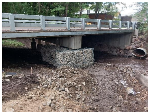
Gabion Basket Mitigation Protects a Bridge Structure
